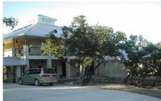
Wireless Internet mounted on the top roof
